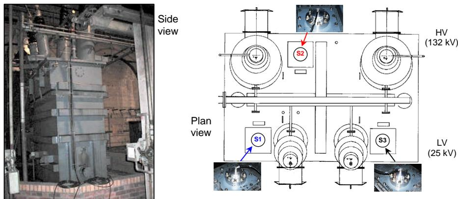
Figure 11: An 18 MVA Single Phase Traction Transformer Equipped for UHF Monitoring
