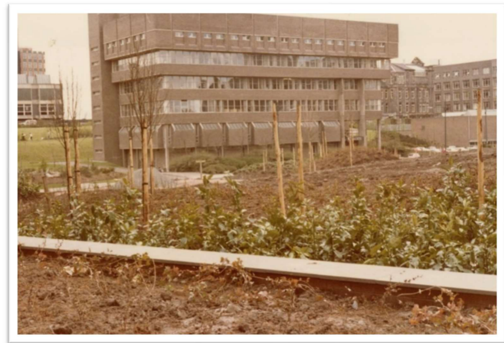
The Law School moved into the Stenhouse Building in 1972-1973 and remained there until 2006 when it moved to the Lord Hope Building. Photograph of the Stenhouse Building, 1980. University of Strathclyde Archives and Special Collections, reference OP/2/4/22.
