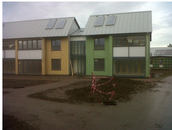
Figure 3 Apartment block (monitoring site)
