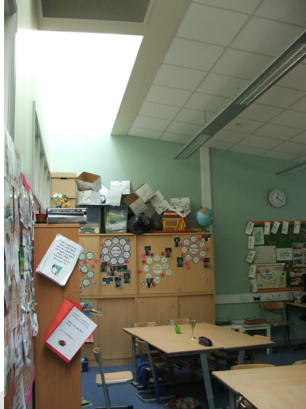
Figure 2: Image showing skylight in interior wall of classroom
