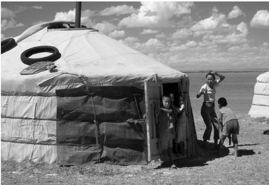
The felt covering for the roof and the lattice walls can be clearly seen; the front door is on the right hand side.
