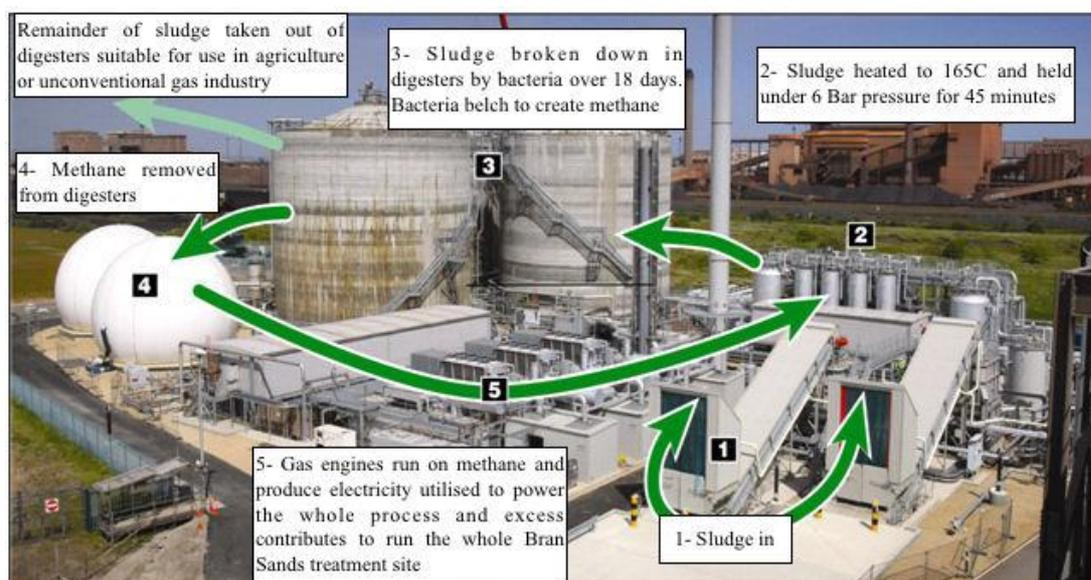
**Figure 1.** Schematic diagram of advanced digestion plant. Modified from North East Bioresources & Renewables (NEBR) (<http://www.nebr.co.uk/>).
