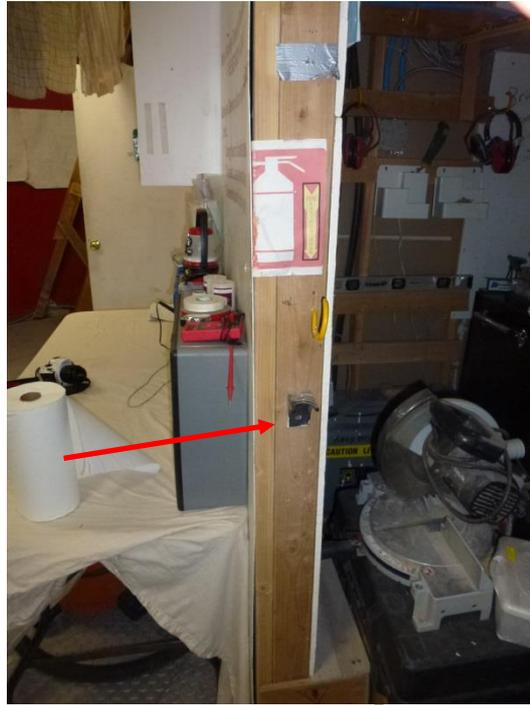
**Figure 5 Damaged fire extinguisher bracket on the MDRS**
