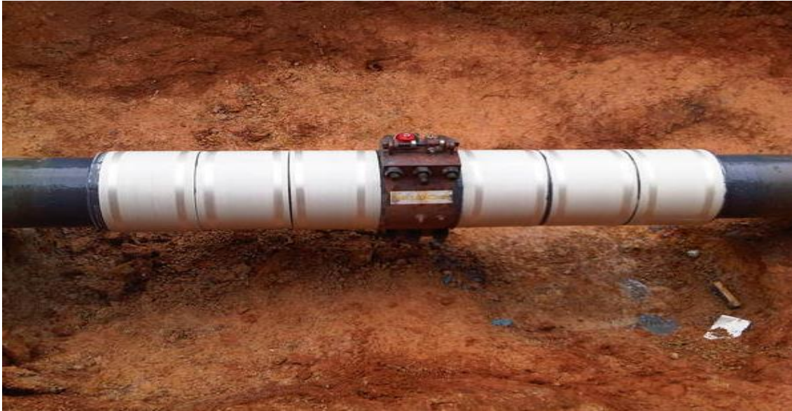
Figure 10. Crack repair using crack arrestors [163]
