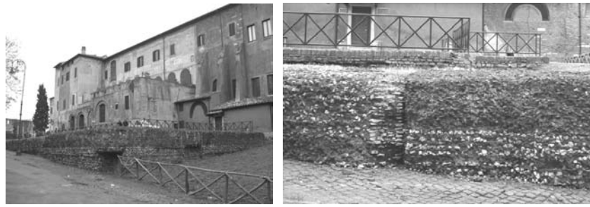
Figure 7: NW corner of the platform a) General view b) Detail
