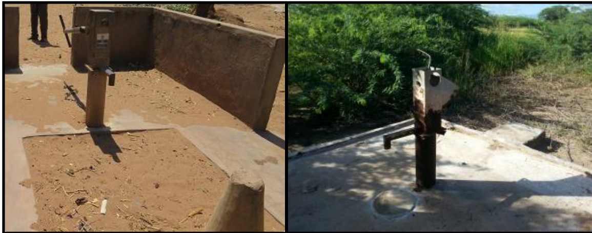
Figure 3. Photograph of a rural water supply that has been deemed a Stranded Asset due to poor borehole yield ( left ) and a rural water supply stranded due to poor water quality ( right ).
